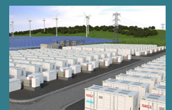
Renewable energy plant with stationary storage batteries
